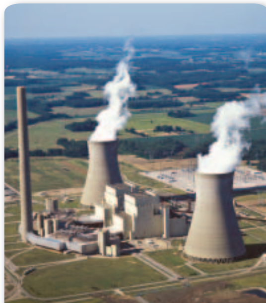
■ Figure 18.10 Sulfur trioxide, a waste gas from the burning of coal, can be removed from smoke-stack gases by combining it with magnesium oxide in a Lewis acid-base reaction. Note that while there is a good deal of steam coming from the cooling towers, there is little visible smoke from the smokestack.
